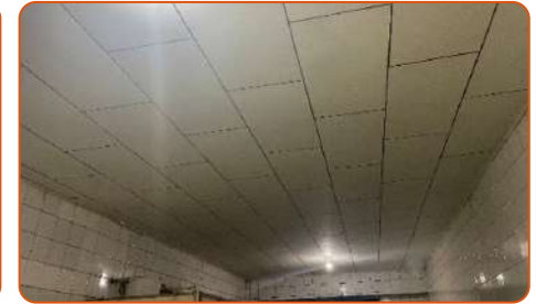
Corrective Action: Light bulb replaced.
