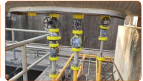
Corrective Action: Leak inspection conducted and sealant tape replaced.
