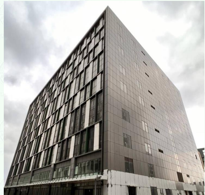
Taoyuan Aerotropolis Free Trade Zone Value-Added Building F10 Project (Completed in March 2023)
