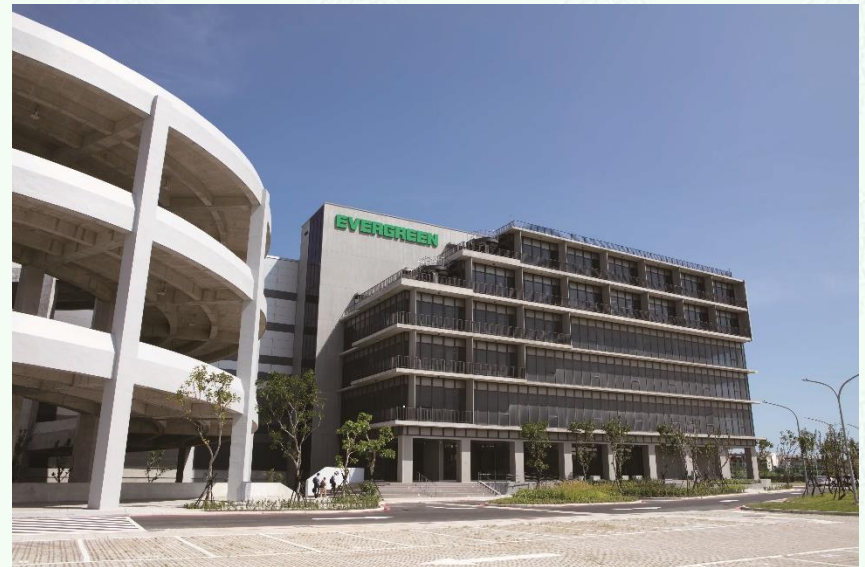
Evergreen International Storage & Transport Corp.'s Dayuan Logistics Park (Completed in January 2023)
