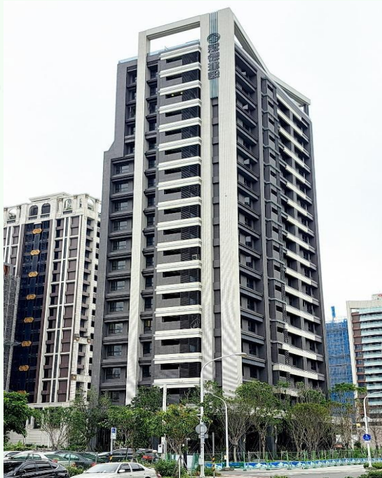
Kindom Construction's F Construction Project in Sanchong (Completed in January 2023)
