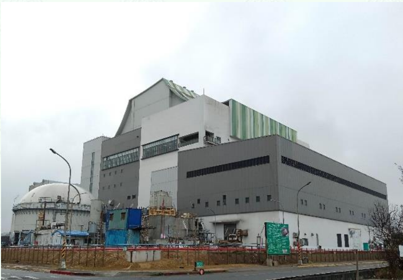
Biomass Energy Center BOT Project (Completed in January 2023)
