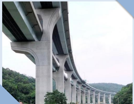
Steel structures of the Taishan-Linkou Section of the Wugu-Yangmei Overpass
